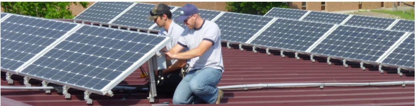
Solar panels being installed at Harcourt Church
